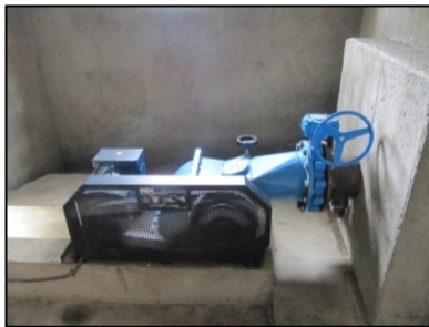
Figure 1.2 Banki turbine and generator – Dump loads
